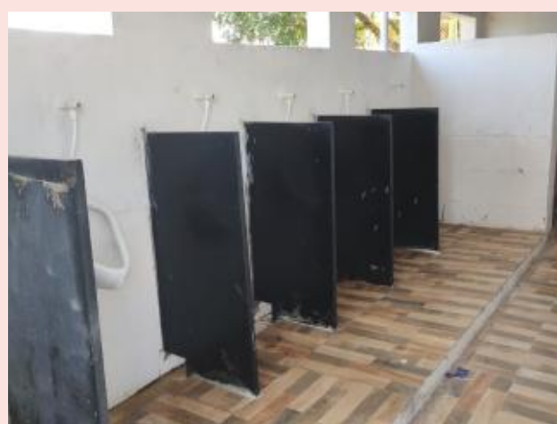
Construction of School Toilets: In 4 Govt. Schools of Gangapur block of Aurangabad District, 7 toilet blocks for boys and 25 toilet blocks for girls were constructed. With a view to ensuring the continual availability of water, CF has constructed 6 water tanks in Gangapur.
